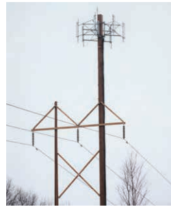
Joint-use structures
